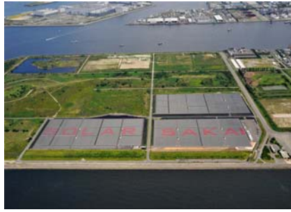
Photo 5-1 The Sakai Mega Solar Power Plant
